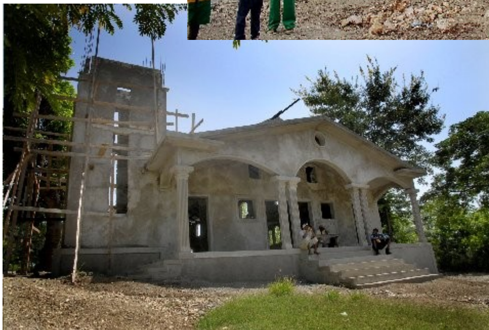
Church pres- ently under construction in Tierra Mouscady, Haiti
