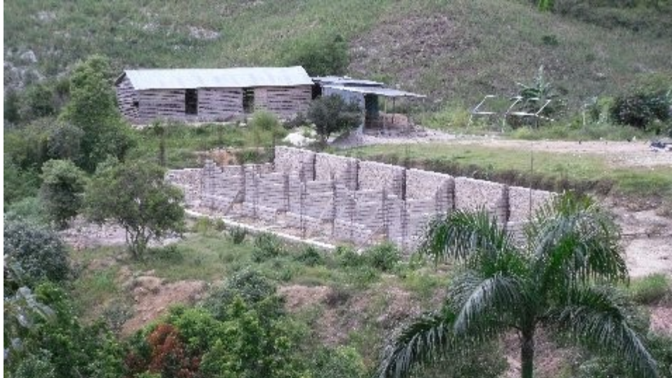
La Pleiade Community School in Cange, Haiti, under construction.
